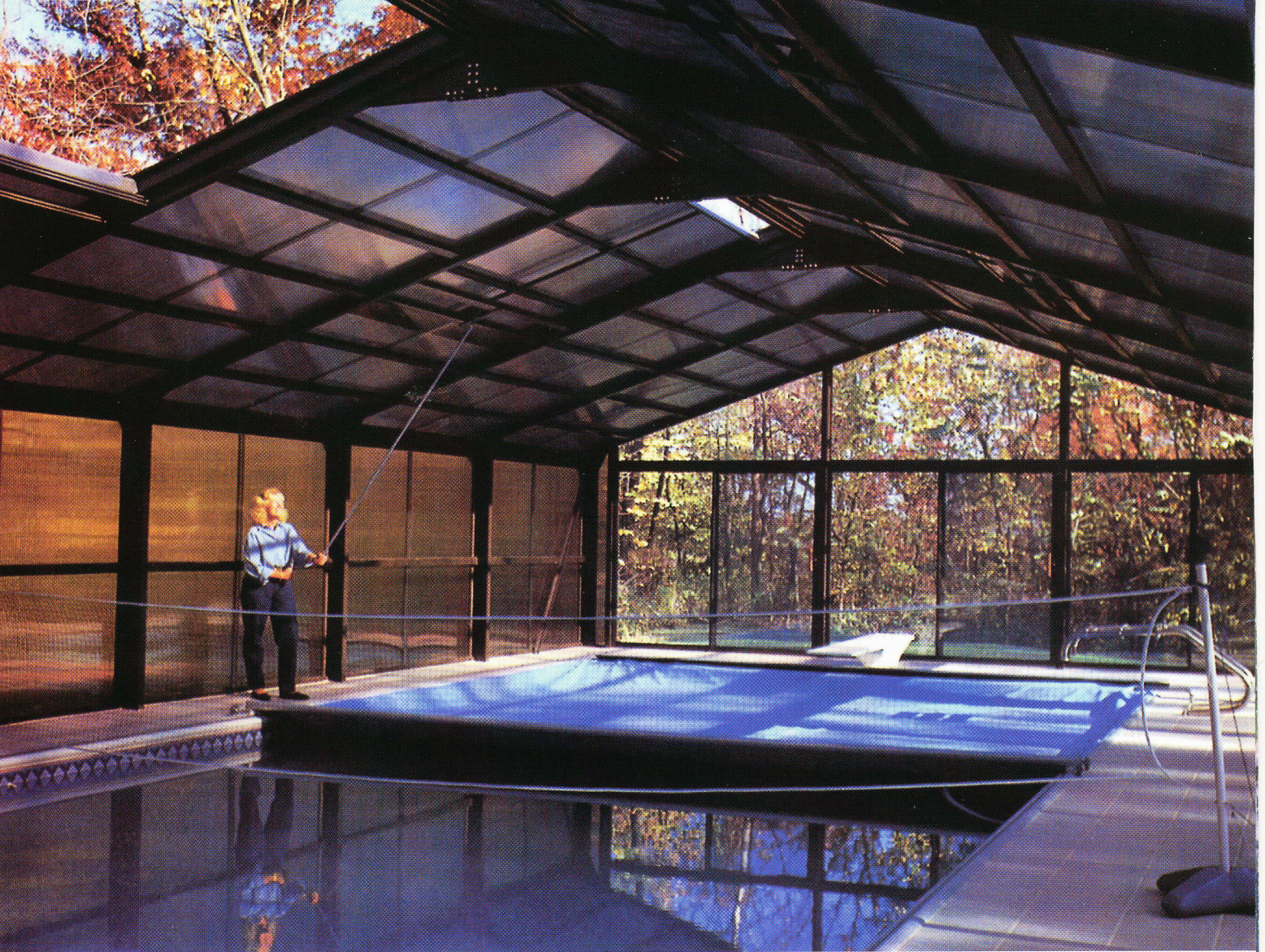
By opening ceiling panels with a crank, Vita avoids possible mechanical failures.
